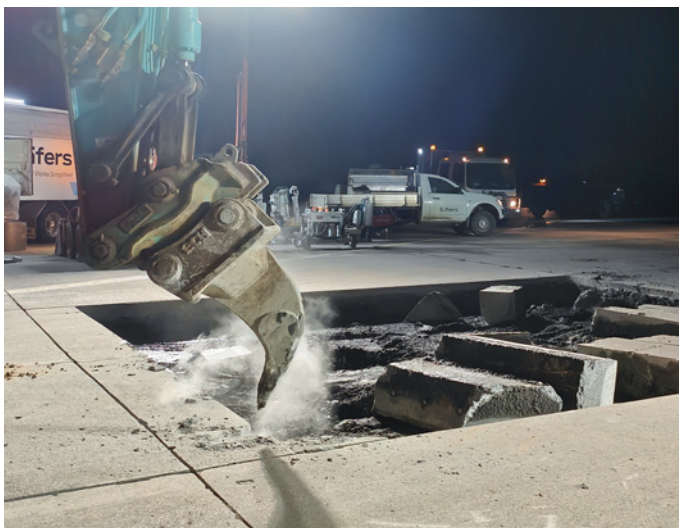
Demolition of existing slabs (7.6 × 7.6 m)
