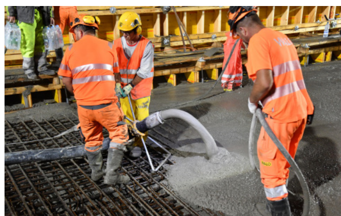
Pump mix used on bridge trough
