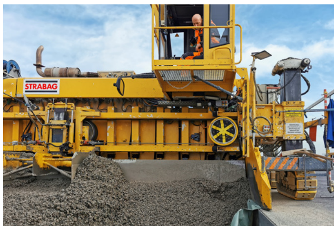
Feeding of the concrete paver with Concretum® Q-FLASH 2/20
