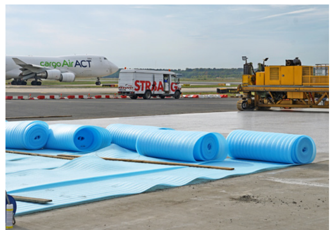
Curing of the finished concrete slabs while aircrafts are operating
