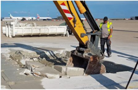
Breaking out existing slabs and removing old concrete
