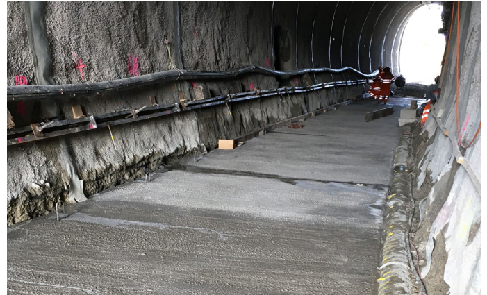
renewal of railway tunnel base - "Russentunnel"
