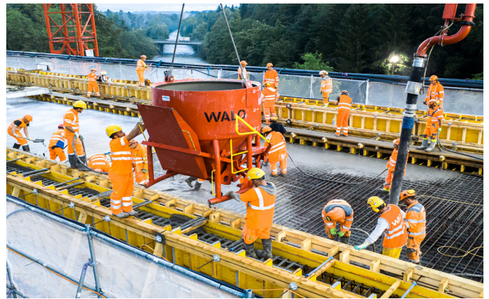
casting of railway bridge deck - "Senseviadukt"
