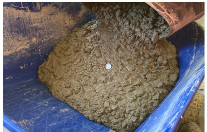
Concrete trials before production
