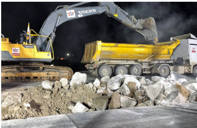
Demolishing existing concrete slabs.
