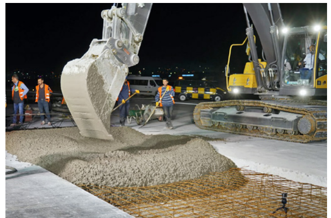
Fixing reinforcement, unloading and spreading the concrete evenly.
