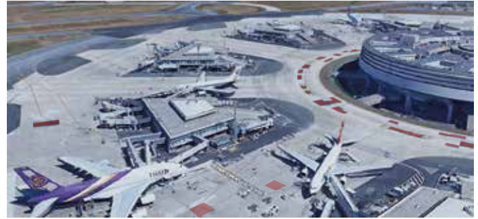
Figure: Damaged spots/areas in the apron/stands area
